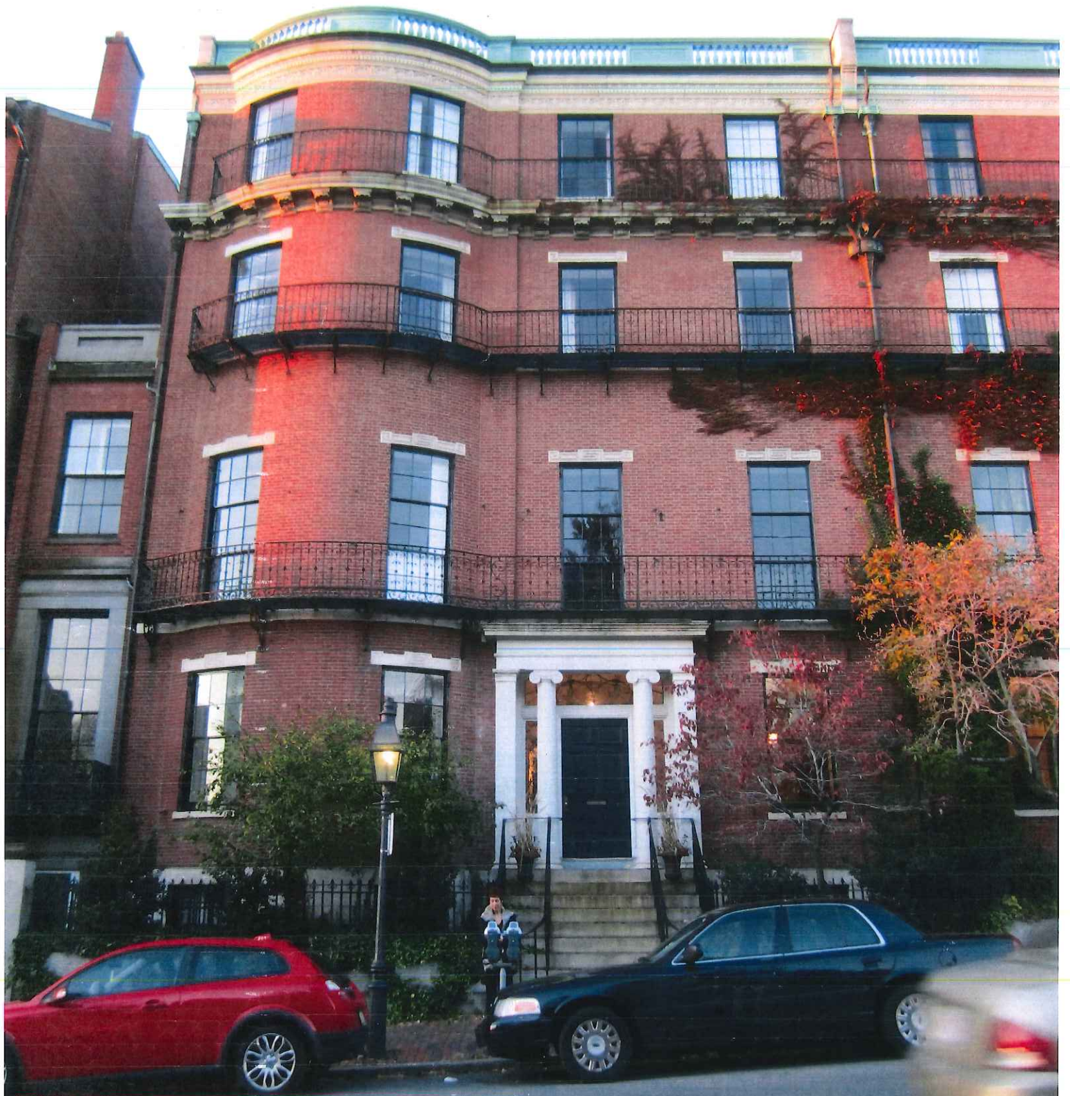
EXISTING 40 BEACON ST. (FROM SIDEWALK ACROSS BEACON ST.) 05.15.17
