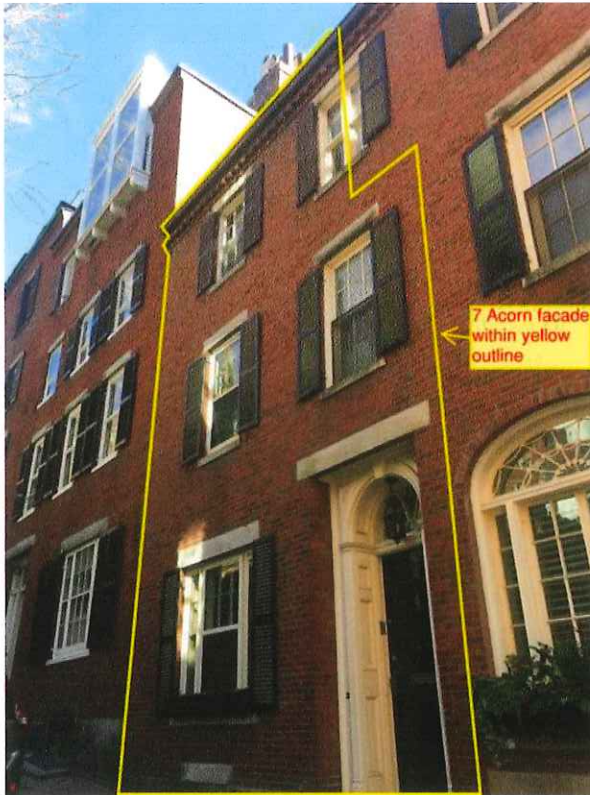
Front façade visible from Acorn Street
