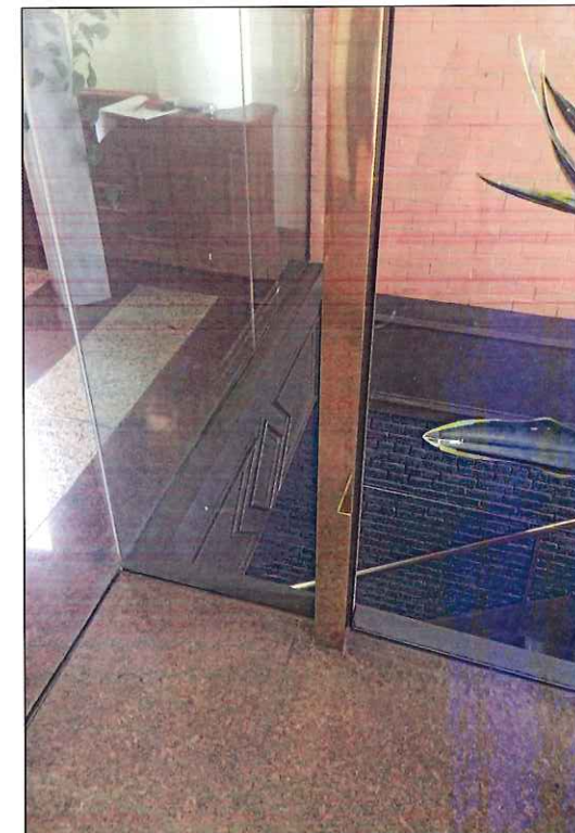
threshold condition @ interior vestibule
