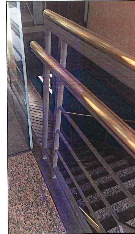
existing guardrail / handrail configuration
