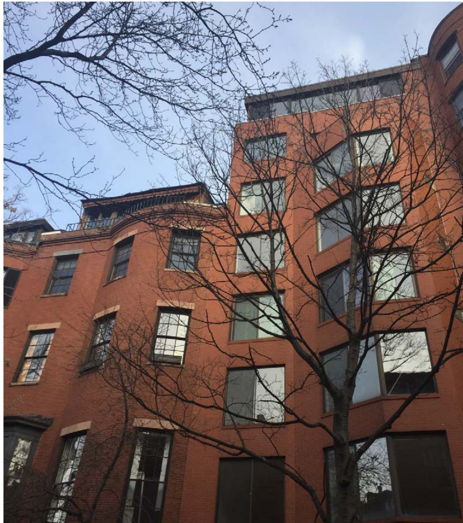
Front Sightline Looking North Existing
