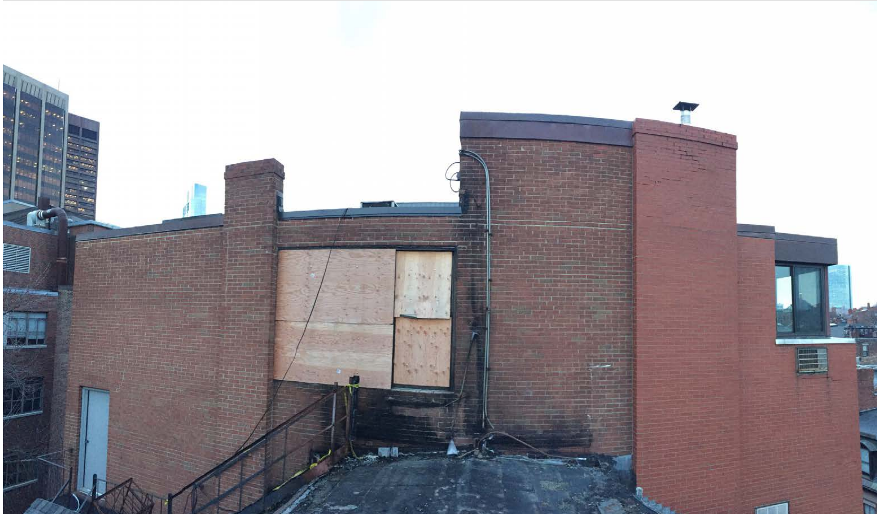
34 Hancock Street Unit 8A Roof and Fire Escape Access Condition
