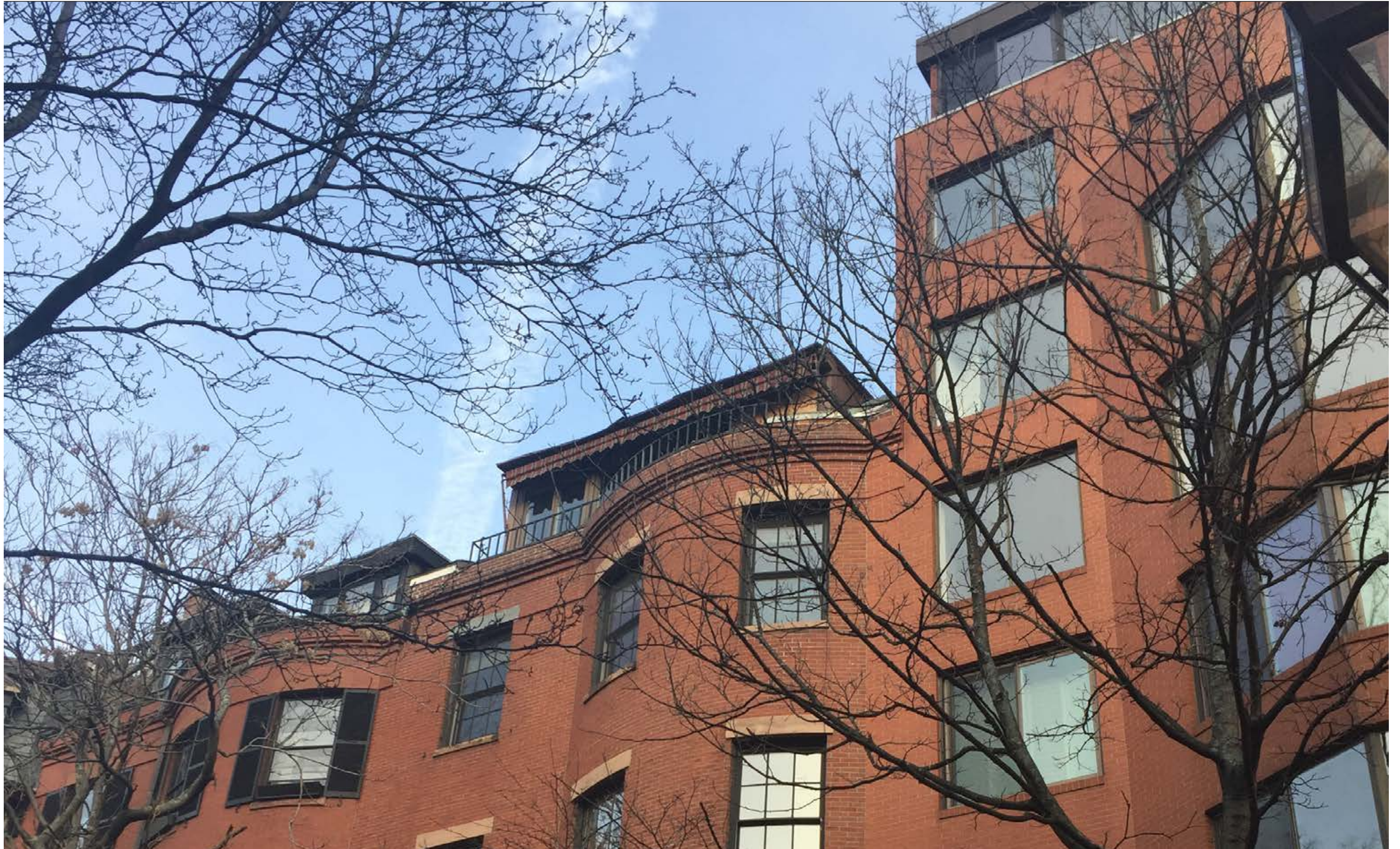
32 Hancock Street Front Dormer
