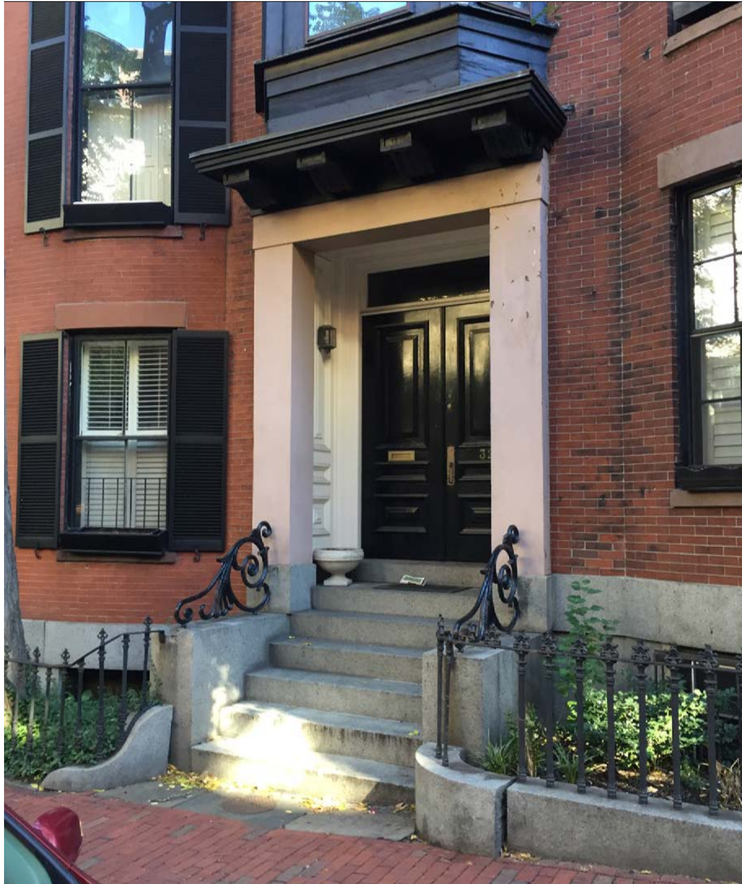
32 Hancock Street Front Entry
