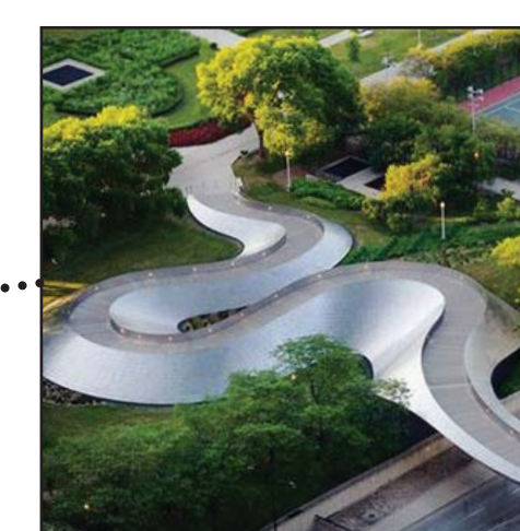
MONUMENTAL PEDESTRIAN BRIDGE
