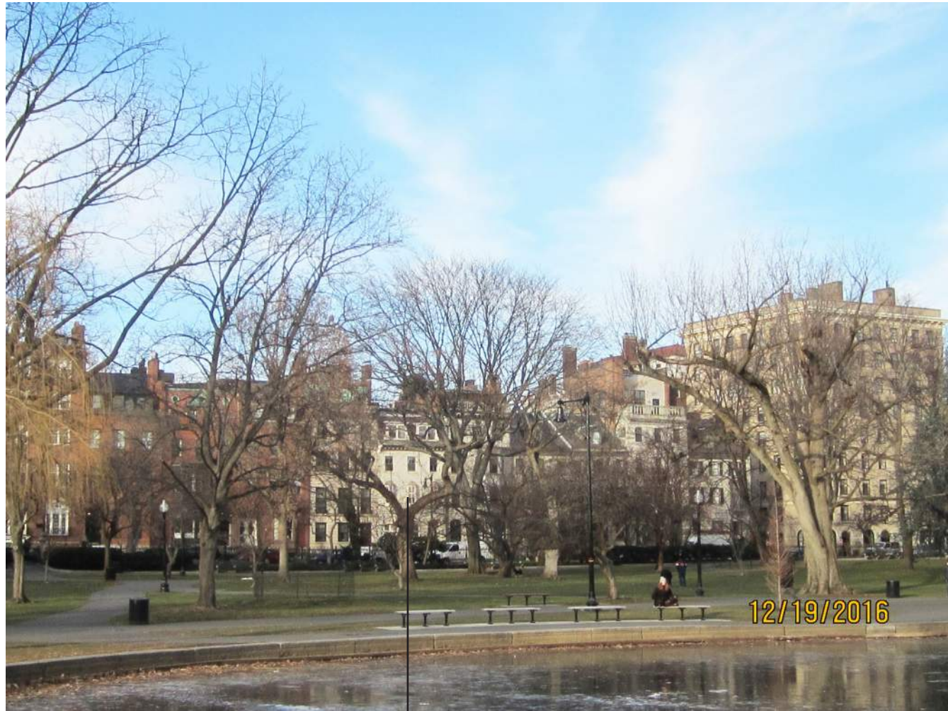
75 Beacon street existing facade
