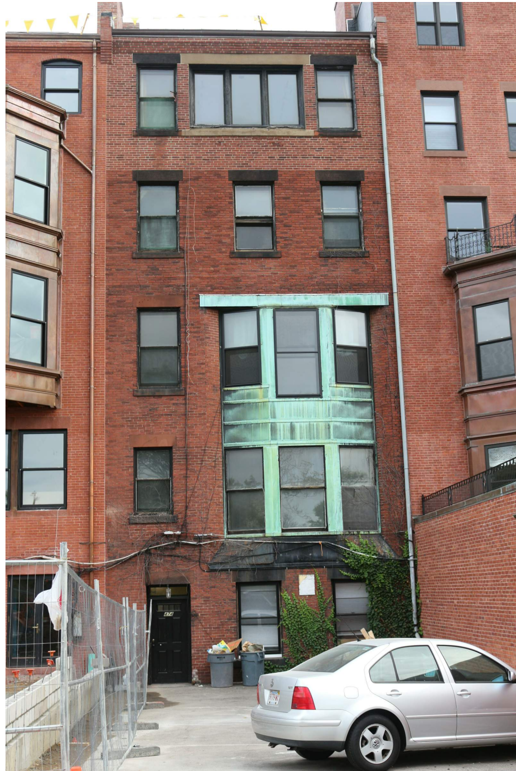
EXISTING CONDITIONS AT REAR PARKING WITH 472 BEACON CONSTRUCTION UNDERWAY
