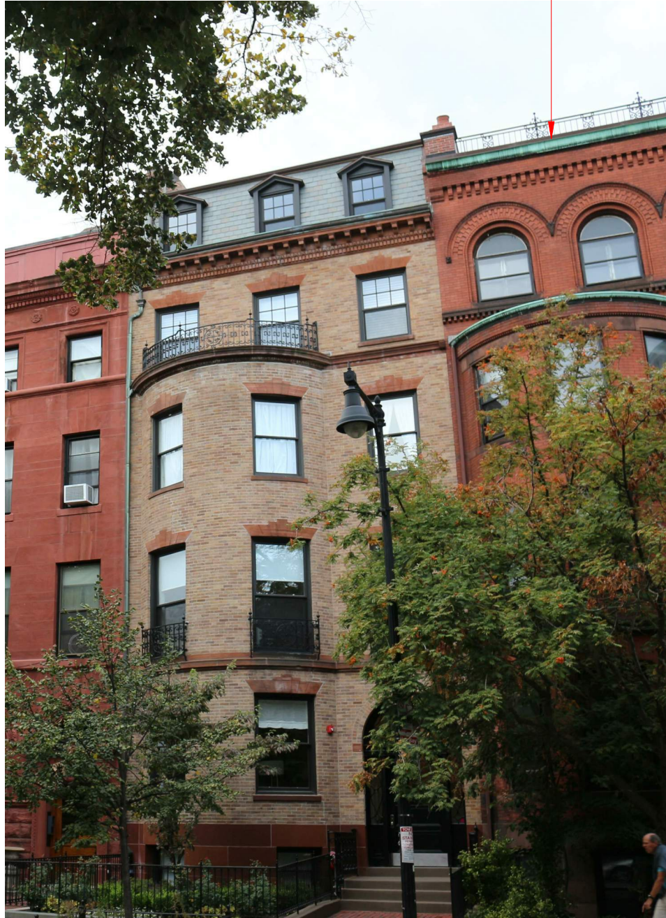
ABUTTING PROPERTY - 476 BEACON STREET
