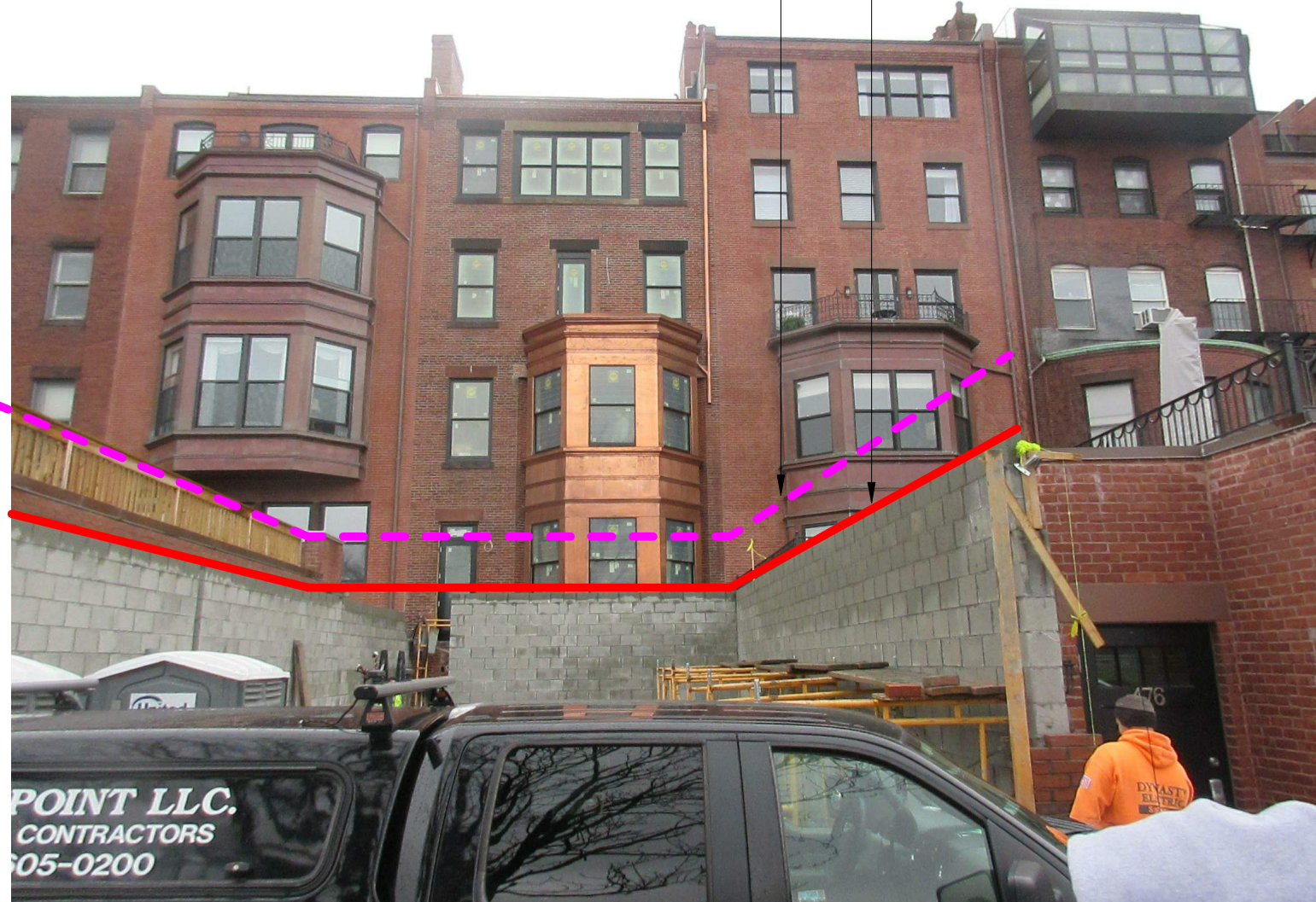
GARAGE CONSTRUCTION AS VIEWED FROM BACK STREET
