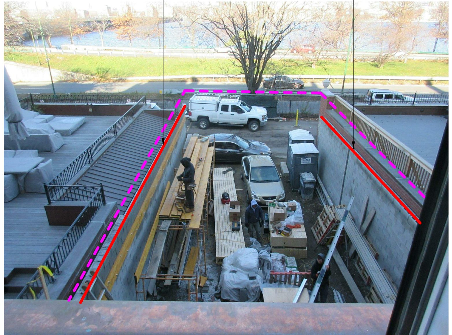
GARAGE CONSTRUCTION AS VIEWED FROM BUILDING'S SECOND FLOOR
