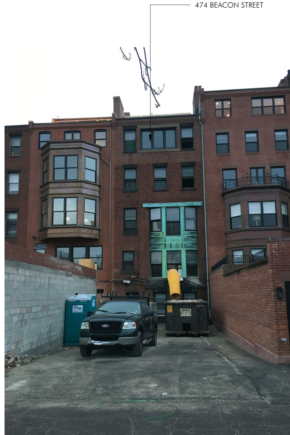
EXISTING CONDITIONS AT REAR PARKING ADJACENT GARAGE EXTENSIONS CONSTRUCTED
