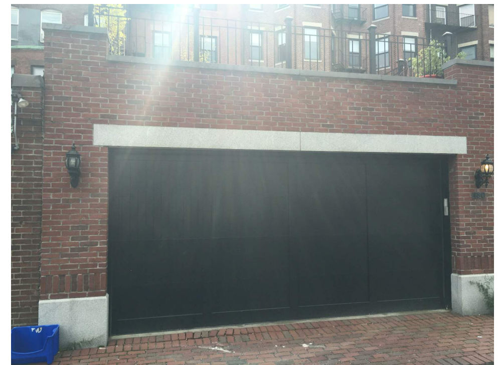
REAR GARAGE WITH ROOFTOP DECK AT 480 BEACON
