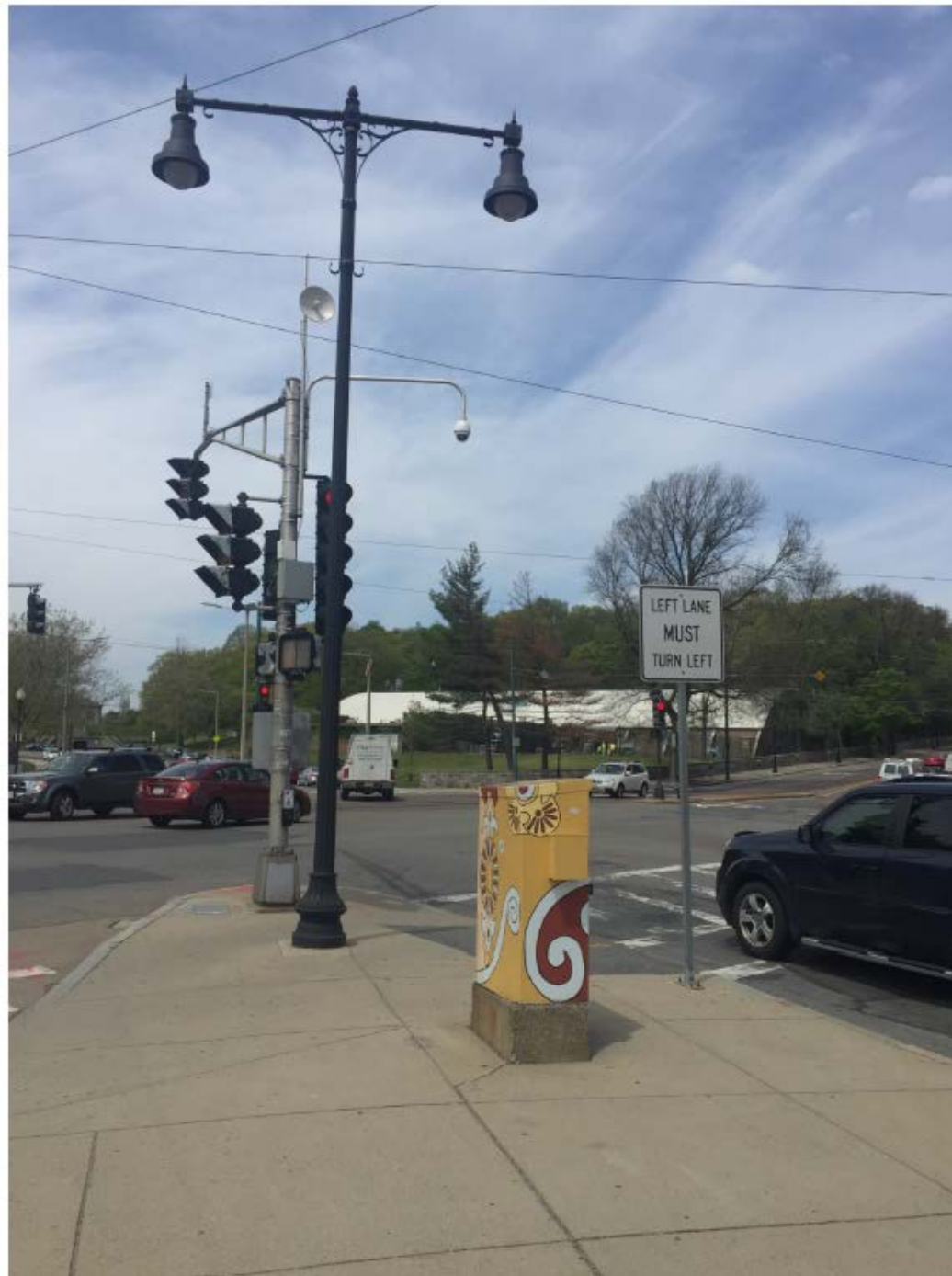
Figure 5 - Traffic Cabinet to be Retained
