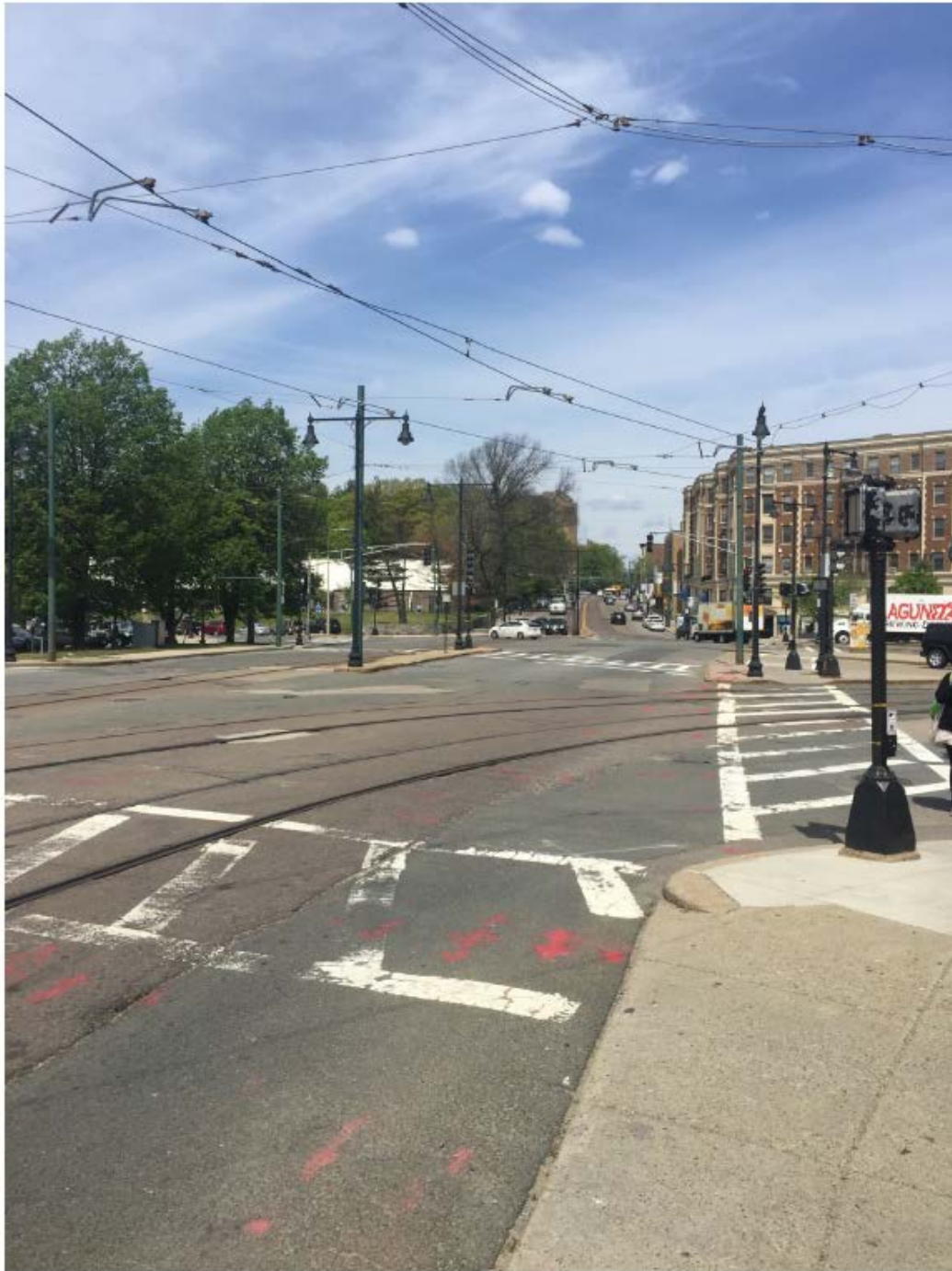
Figure 1 - Near-side Pedestrian Signal Post, Base, Foundation and Head to be Replaced (Typ)
