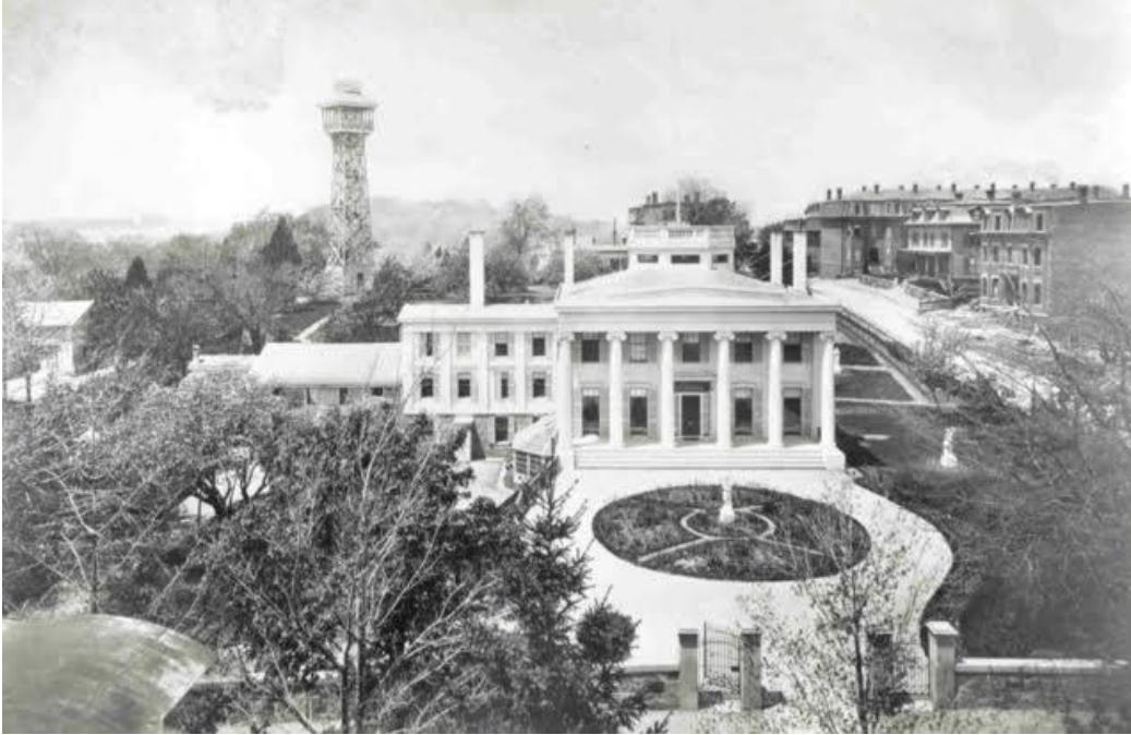
9. Kittredge House property, view to west, 1880s. Bradlee's observatory tower at upper left; Linwood Street on right.
