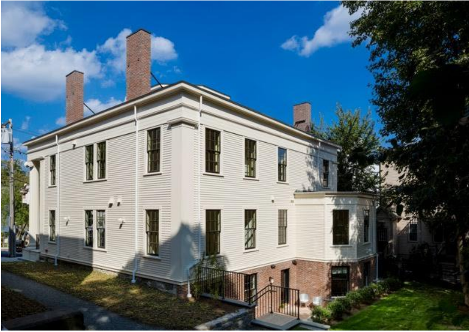
3. West and south façades (Photo by Greg Premru, 2014).
