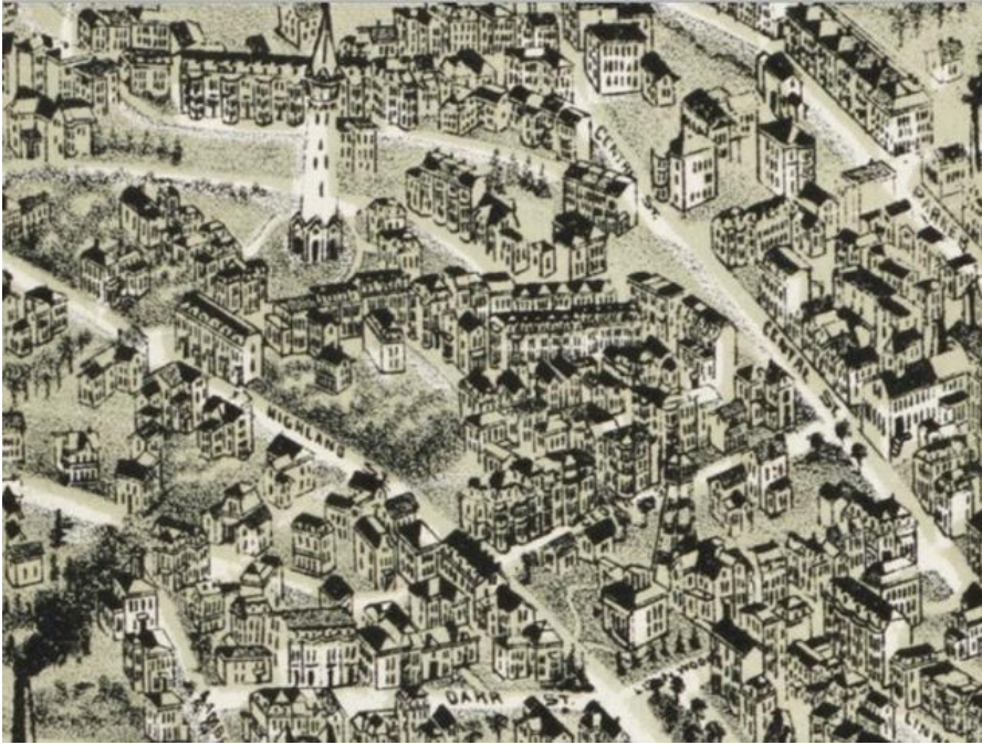
7. Bird's eye view of Roxbury Highlands, looking southwest, 1888. Cochituate Standpipe at upper left; Alvah Kittredge House at lower right.
