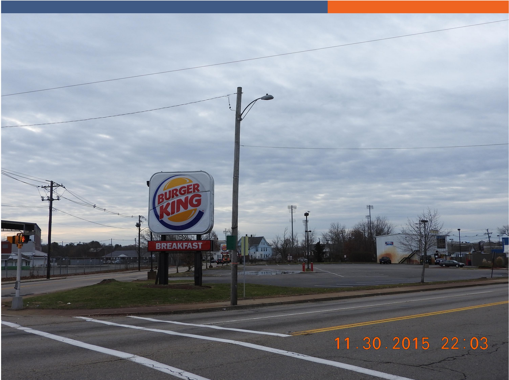
Existing Conditions: Wood utility pole.
