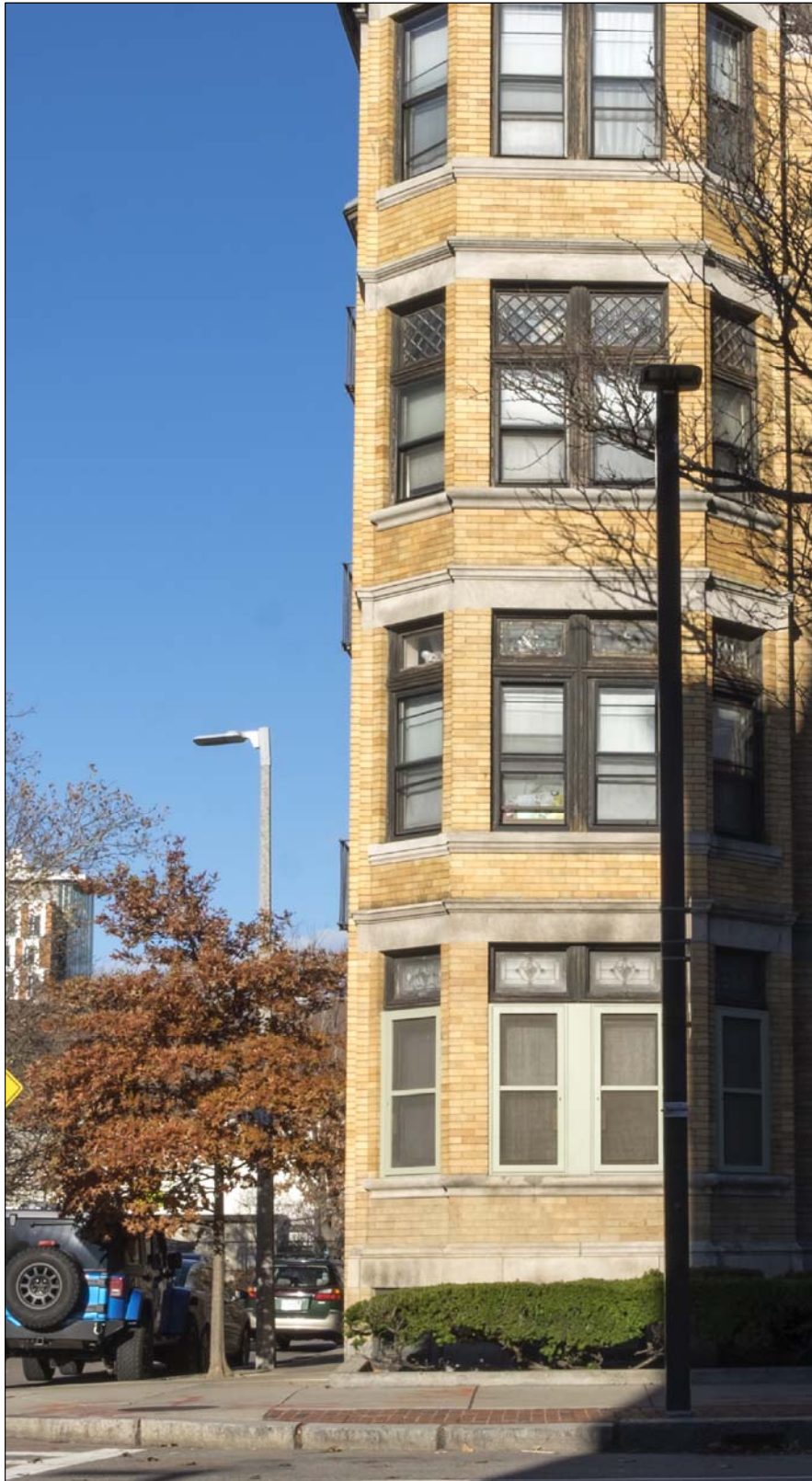
SQUARE CONTEMPORARY LIGHT POLE - AERIATA LUMINARY FIXTURE EXISTING CONDITIONS PHOTOGRAPH - EXHIBIT X-2
