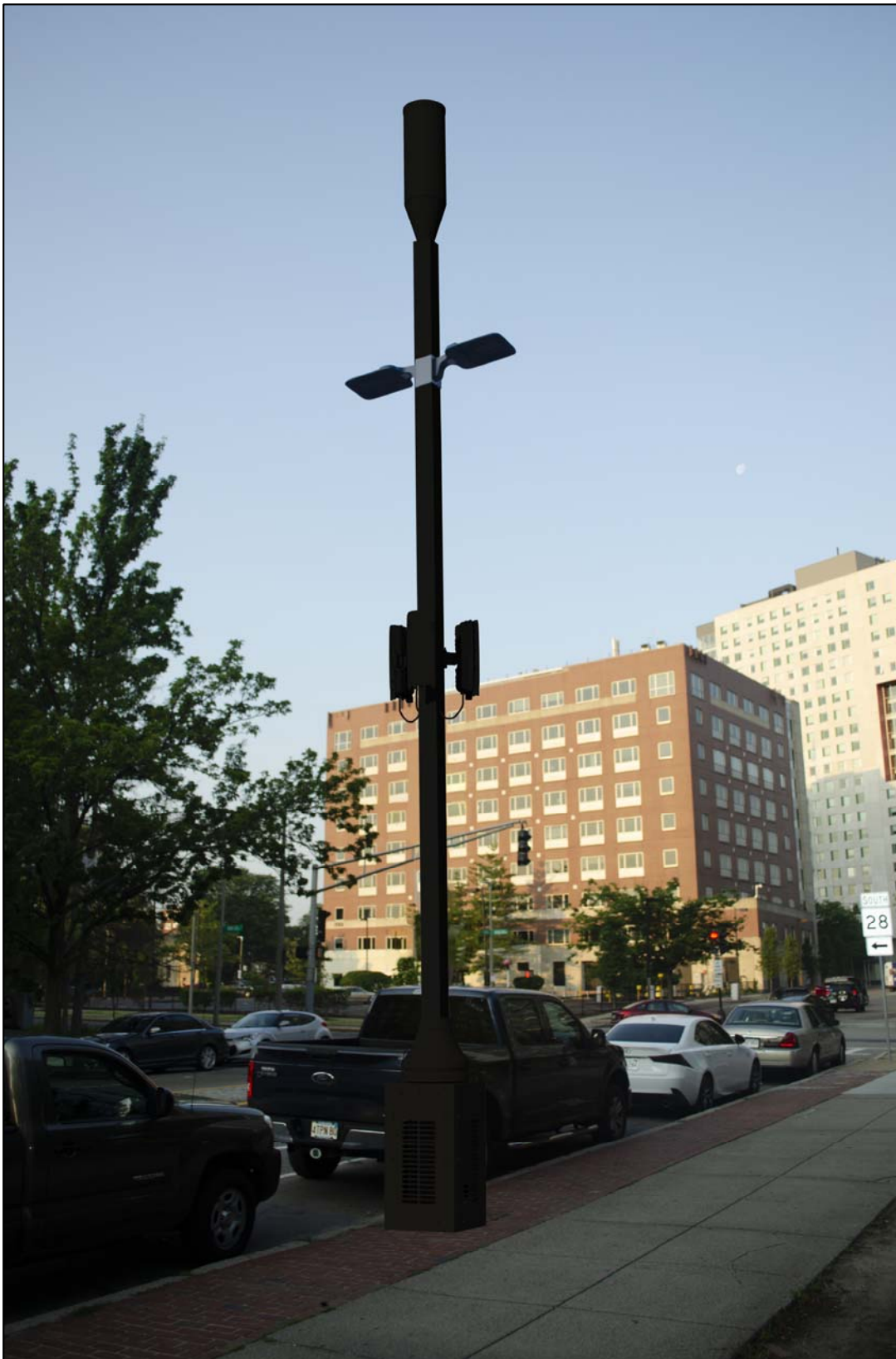
SQUARE CONTEMPORARY LIGHT POLE - DOUBLE AERIATA LUMINARY FIXTURE PROPOSED PHOTOSIMULATION - EXHIBIT X-2B
