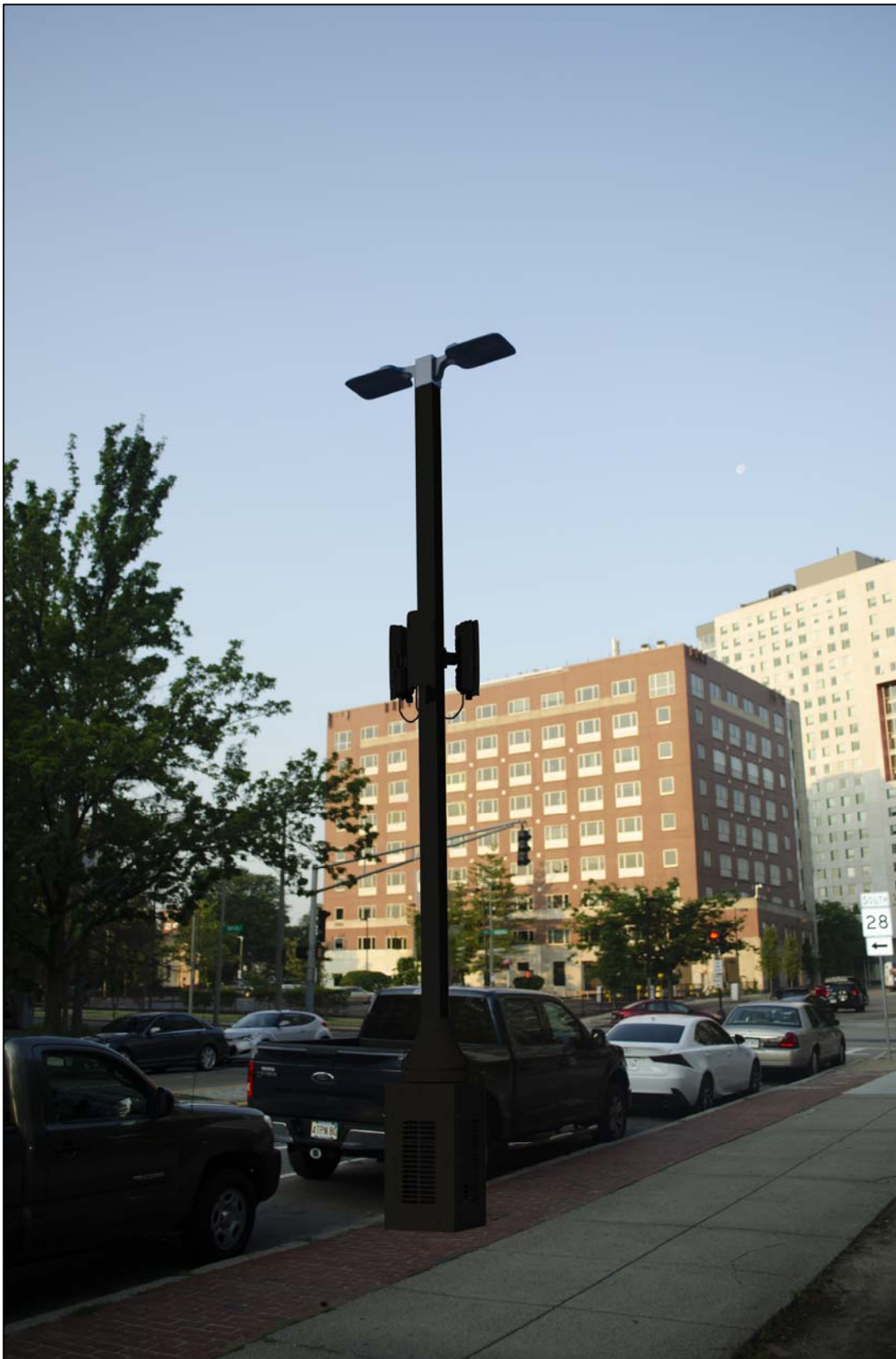
SQUARE CONTEMPORARY LIGHT POLE - DOUBLE AERIATA LUMINARY FIXTURE PROPOSED PHOTOSIMULATION - EXHIBIT X-2D
