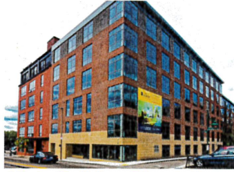
Allele Building Phase II
