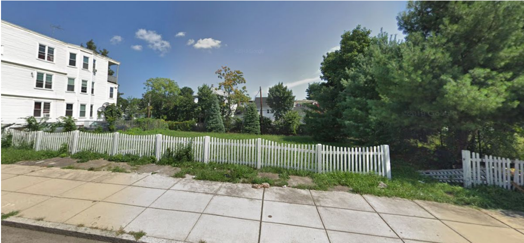
18-24 Standish Street, View from Standish Street
