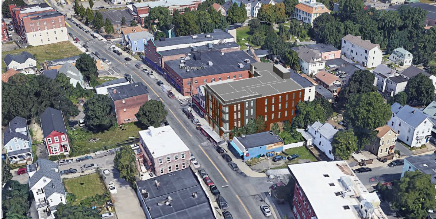
Looking North on Dudley Street
