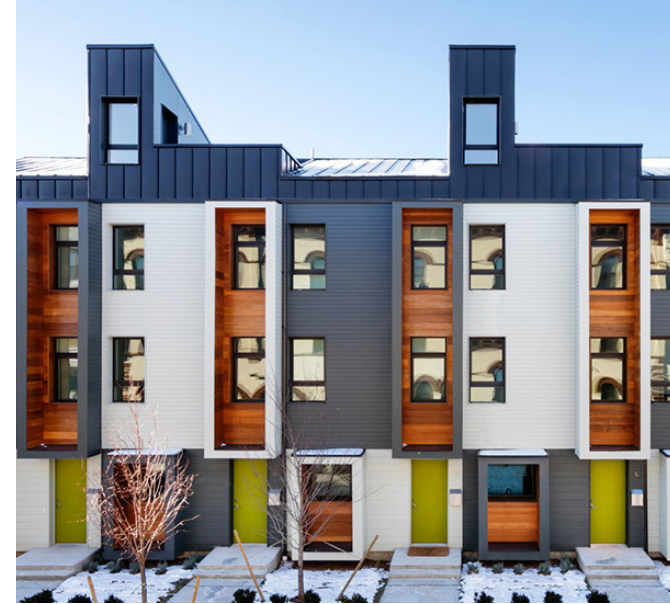
74 HIGHLAND eHOMES 74 HIGHLAND ST, FORT HILL, ROXBURY, BOSTON, MA (Completed)
