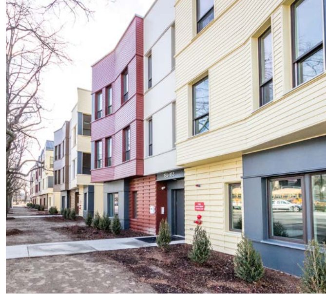
PARCEL U 92 - 171 HYDE PARK AVENUE, JAMAICA PLAIN, BOSTON, MA (Multiphase | Phase 1 Completed)
