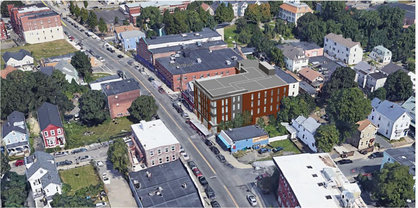
Looking North on Dudley Street
