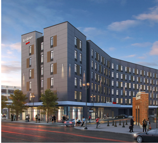
MELNEA HOTEL + RESIDENCES 425-435 MELNEA CASS BLVD, DUDLEY SQUARE, BOSTON, MA (Under Construction)
