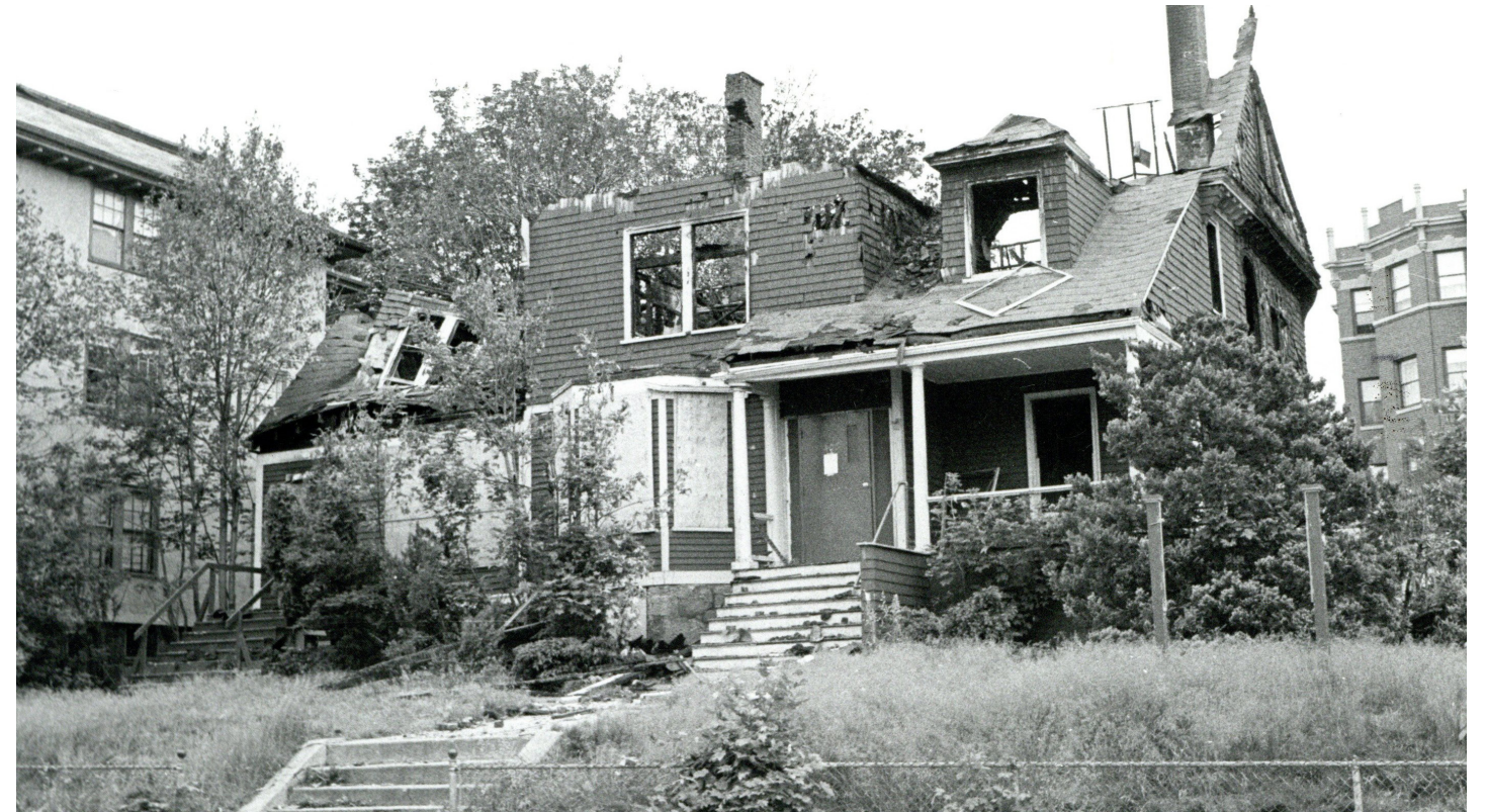
Demolition of former house at 405 Washington Street
