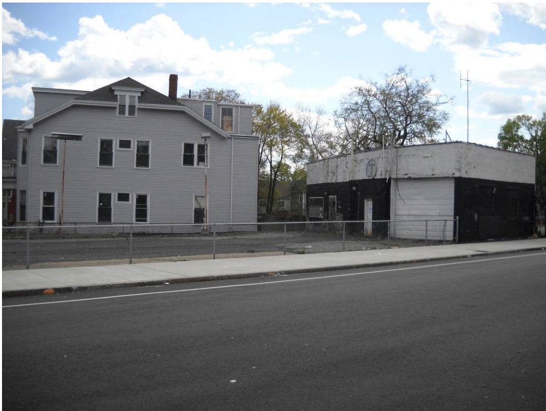
Photograph No. 14: Abutting Former Auto Repair/Filling Station Property Facing Southeast
