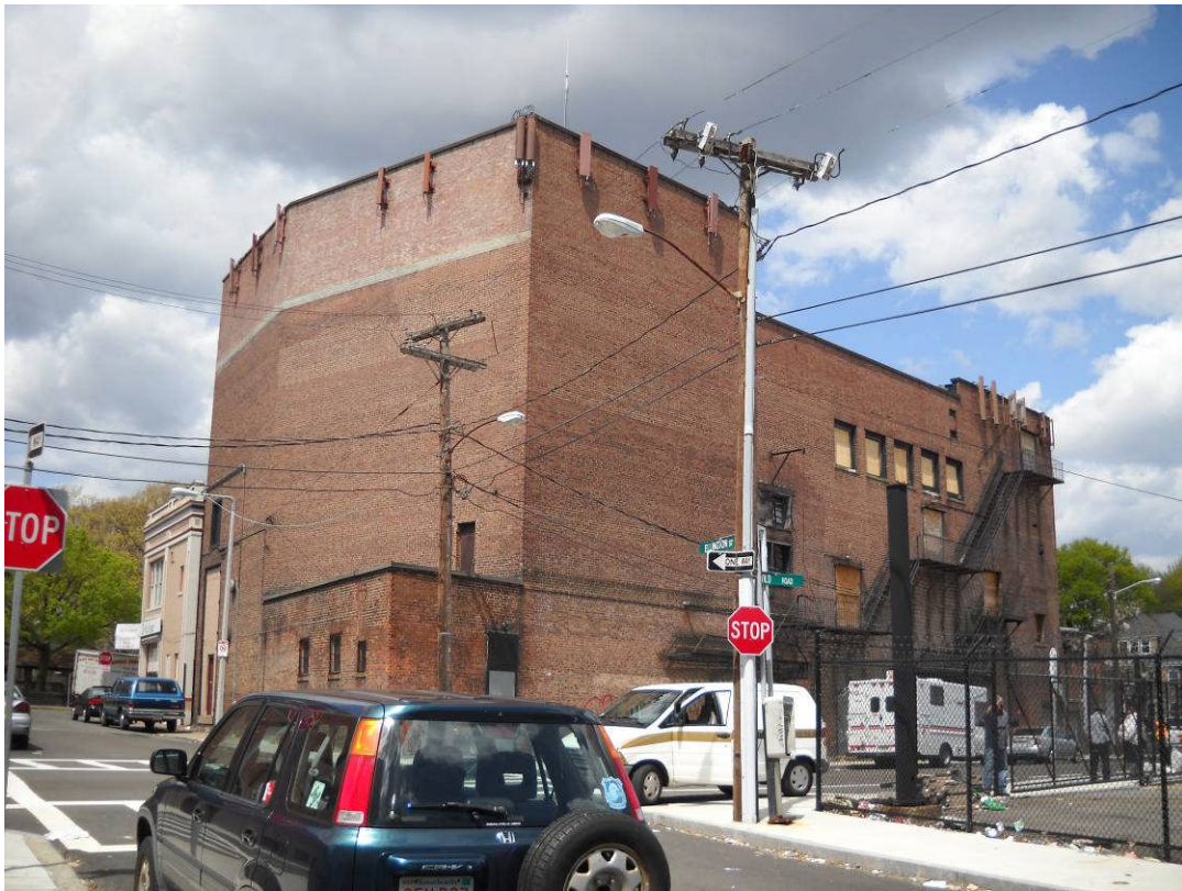
Photograph No. 13: Abutting Church Building Facing Northwest
