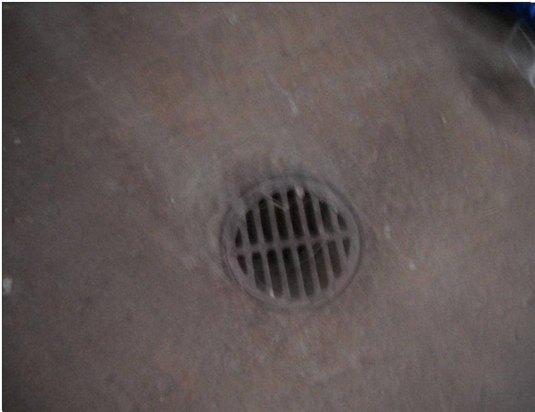
Photograph No. 7: Floor Drain
